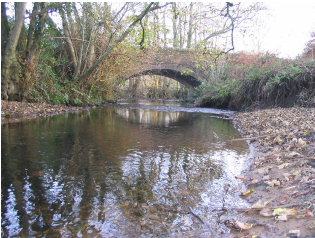
Bideford Brook crossing under Awre Road at Nether Hall Farm
